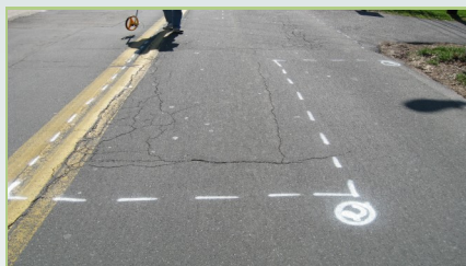
Typical survey paint markings
