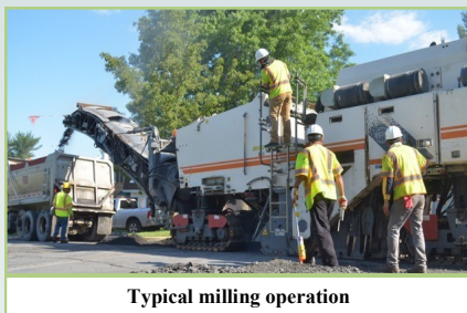
Typical milling operation
